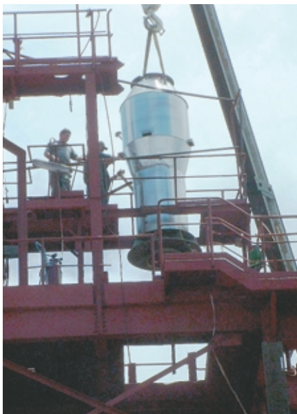
Installation of the oxidation fluid bed roaster.
