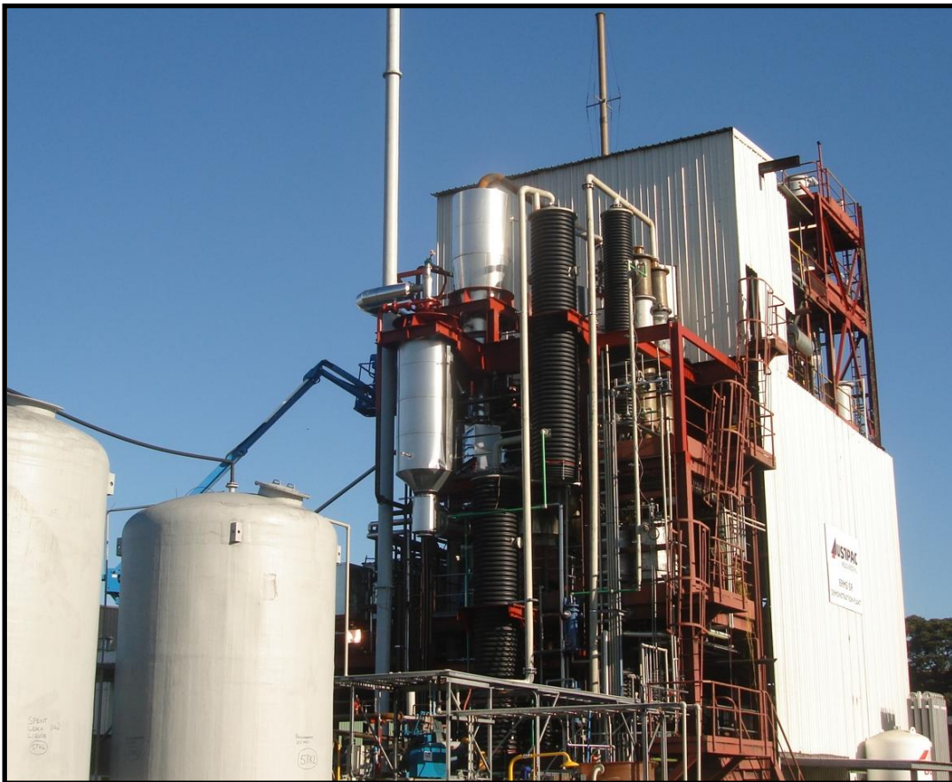
EARS Acid Regeneration Plant
