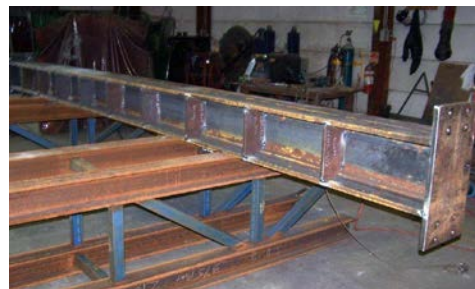
Fabrication of steelwork for tower extensions
