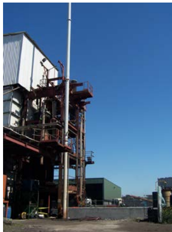
Foundations for north tower extension
