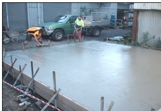
Reinforced concrete slab foundation for briquetter.
