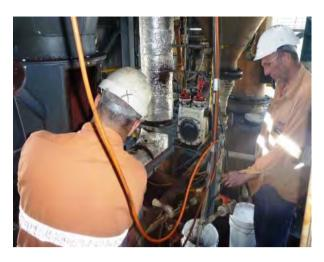
Adjusting slurry feed pump to fluid bed evaporator during pelletising operations
