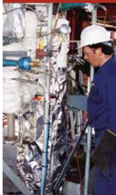
↑ Double dump valve ↓ John Winter operating metalliser
