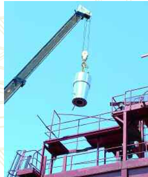
Installation of pre-heater
