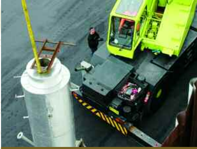
Installation of ERMS afterburner
