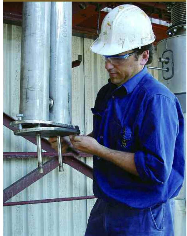
Installation of solids return seal
