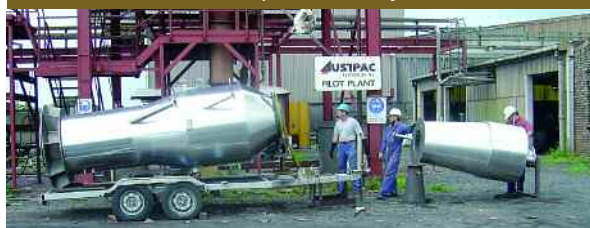
Oxidation roaster and pre-heater ready for installation
