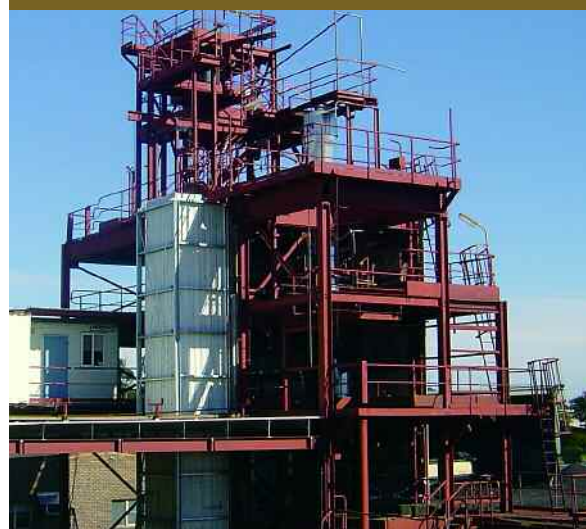
Construction of materials hoist shaft
