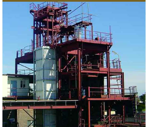
Construction of materials hoist shaft
