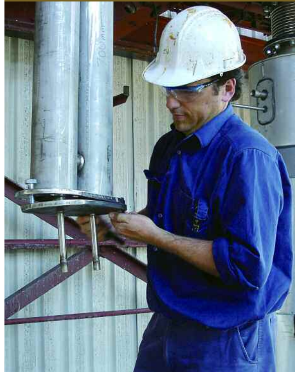
Installation of solids return seal
