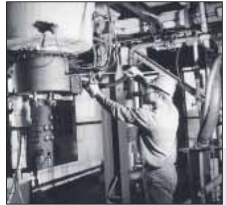
Adjusting combustion air to the large fluid bed reactor
