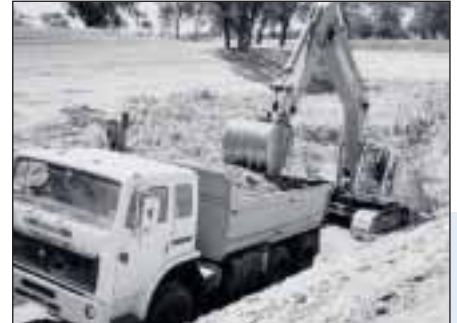
Bulk sampling operations at Drung South
