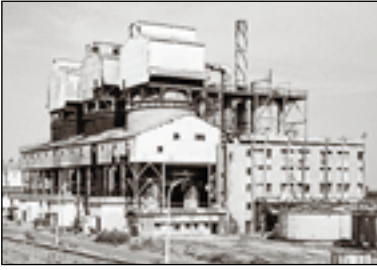
Part of the existing infrastructure at the OSCOM mineral sand processing plant
