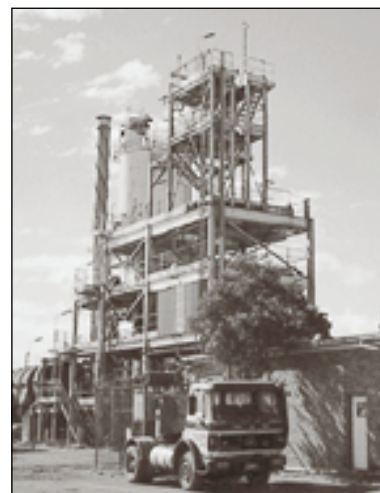
Austpac pilot plant facilities at Kooragang Island, Newcastle
